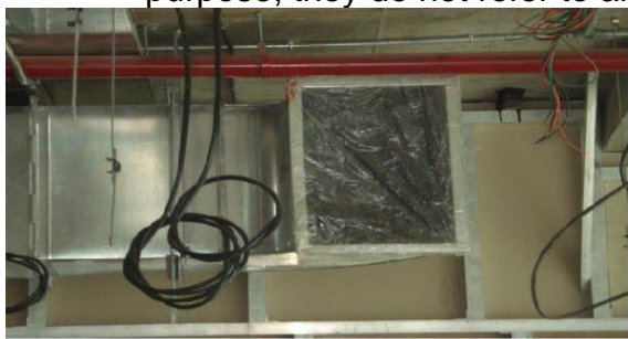
Ducts Wrapped With Plastic To Avoid Dust Ducts Stored with Properly Wrapped with Plastic
